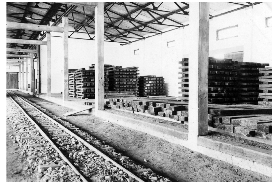
Timber godown showing sleepers stacked for air-drying prior to treatment in wood preservation plant Photo: J.N. Sharma
