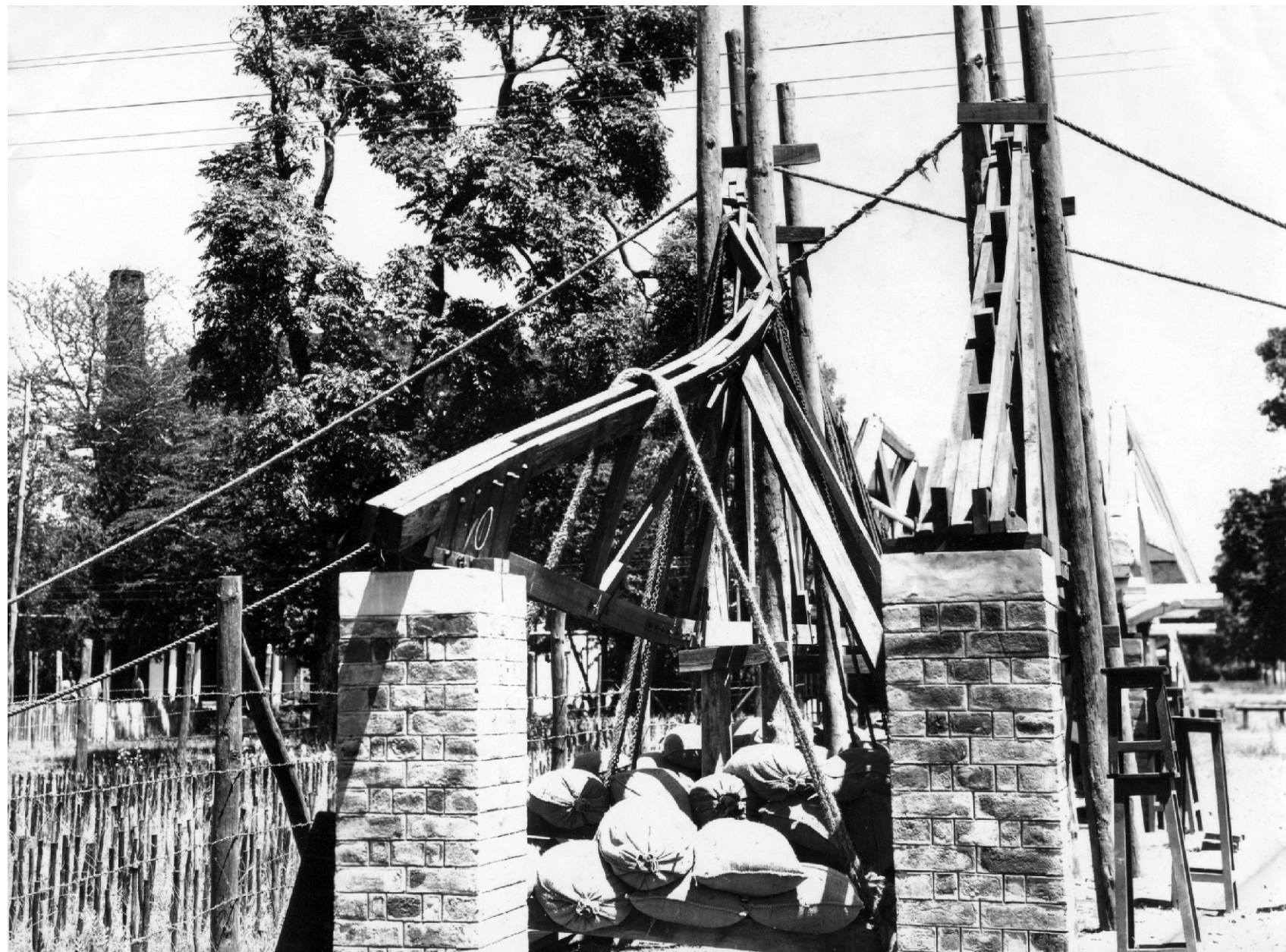
Roof trusses showing the failure of the M.E.S. pattern truss with steel gusset plates and straps. Total load on the truss at failure is only 3½ tons which is only about 75 per cent of the designed load. Timber Testing Section, FRI Photo: V.K. Sharma, April 1942
