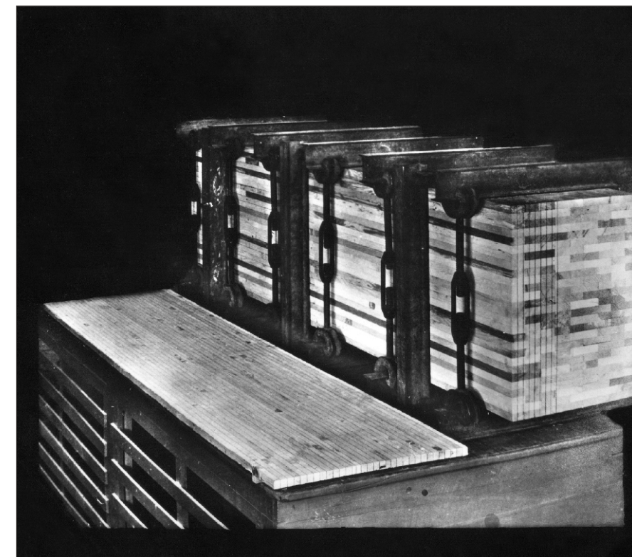
Laminated block being pressed with 'I' beams and retaining clamps, Wood Workshop Section, FRI Photo: M. Bakhshi, 1938
