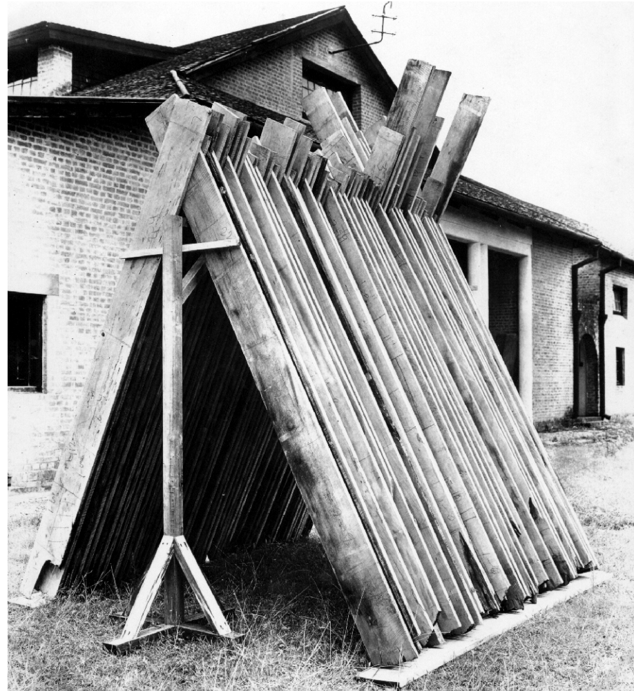
Method of vertical stacking for rapid seasoning (side view), Seasoning Section at FRI Photo: Harswarup, August 1933
