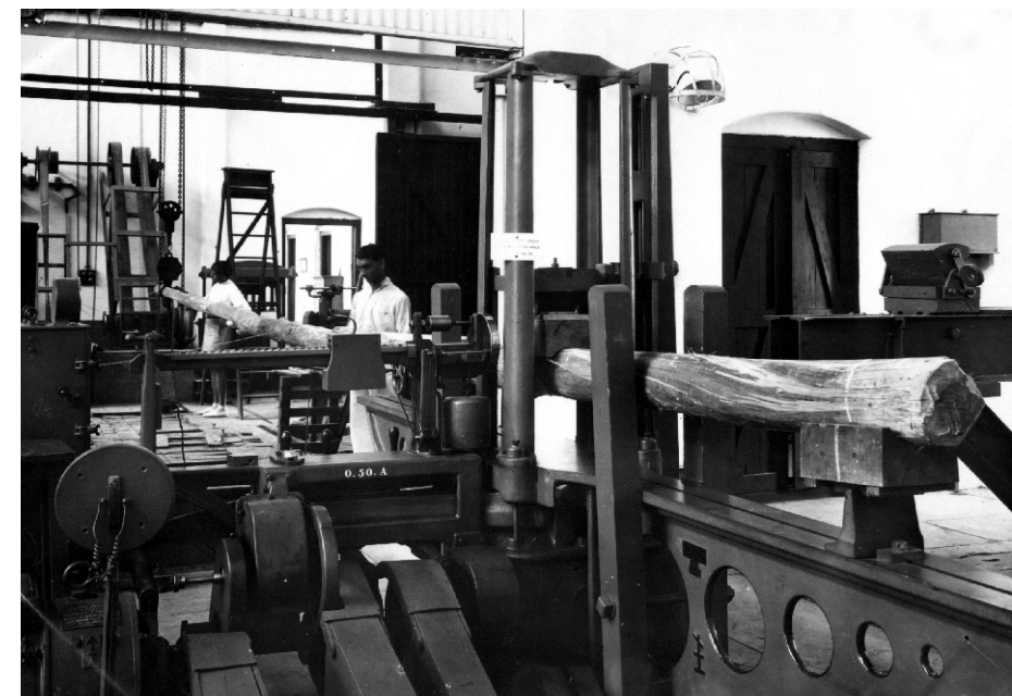
Testing telegraph poles of Shorea robusta , Timber Testing Section, FRI Photo: Harswarup, June 1935
