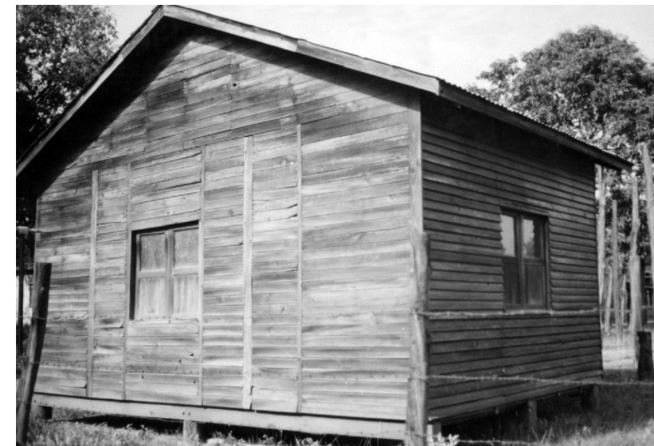
Bamboo hut (1935) treated with world acclaimed ASCU preservative developed in FRI
