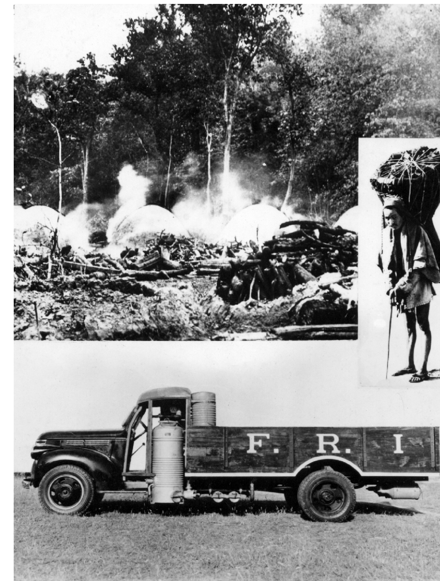
Fuel and charcoal conversion preparatory to burning and planting teak, etc. A coolie carrying charcoal and the FRI motor truck fitted with a charcoal gas plant Photo: V.K. Sharma, June 1942
