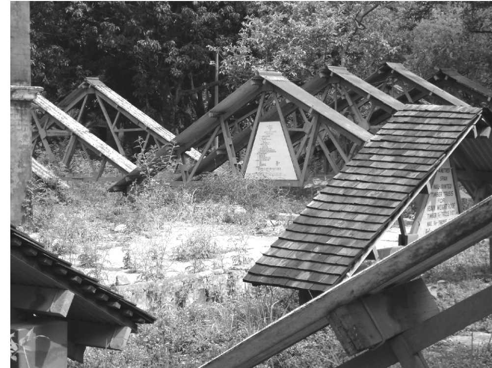
Timber trusses for heavy-weight roofs constructed by Timber Engineering Discipline FRI
